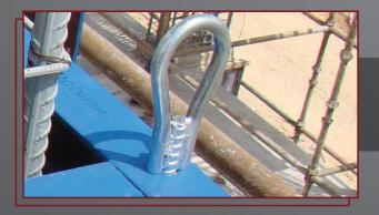
Lifting Hooks act as load bearing points for moving and ensures easy and simple extensions
