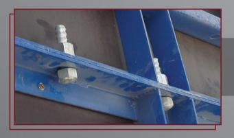
Bolts are used to connect panels together.
